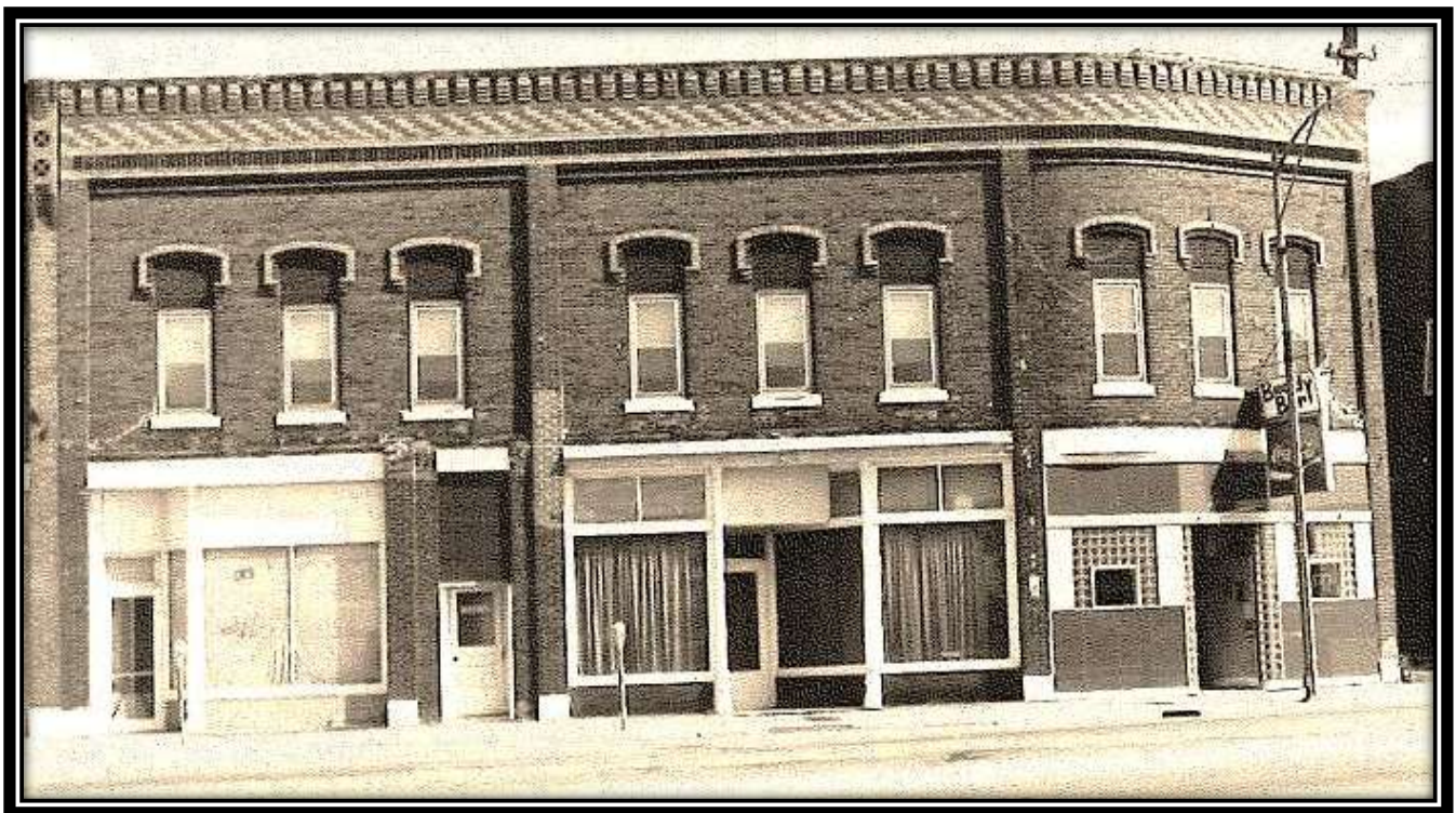
Taken during a State of Michigan Survey in 1975 , the south half of the double building located on the 100 Block of South Stephenson Avenue shows 115 South Stephenson Avenue and other addresses before the remodeling was done for the Brave Bull , Geline’s Rib Cage and Fontana’s Supper Club . [ State of Michigan ]
