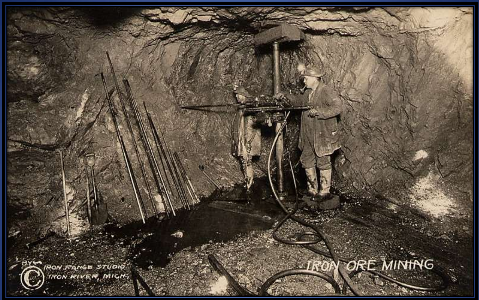
This unused postcard view by the Iron Range Studio, dating between 1920 and 1930, shows two miners using a Rand drill. Note the drill bits lined up against the rock wall, and the air hoses used to supply the compressed air which ran the drill. [WJC Photo]
