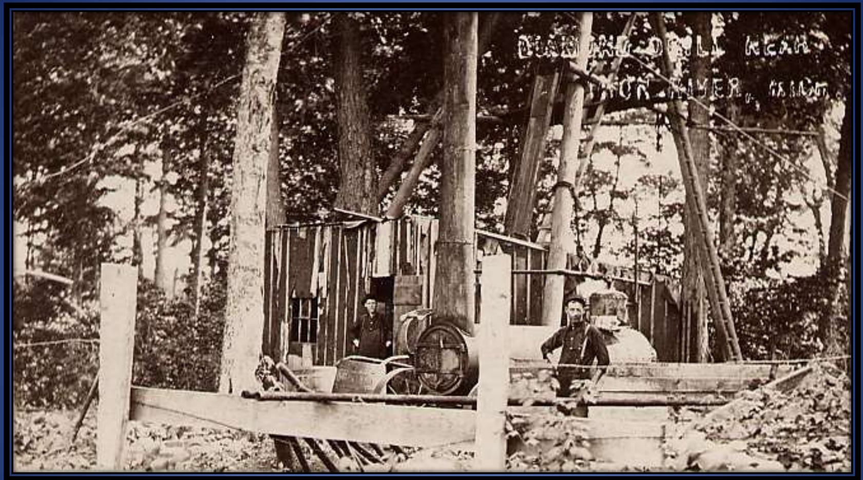
Postmarked August 31, 1912, this postcard view is identified as “Diamond Drill Near Iron River, Mich.” Diamond drilling was done to produce core samples to determine the location of iron ore at various depths. The full height of the diamond drill rig pictured above is not visible. [WJC Photo]
