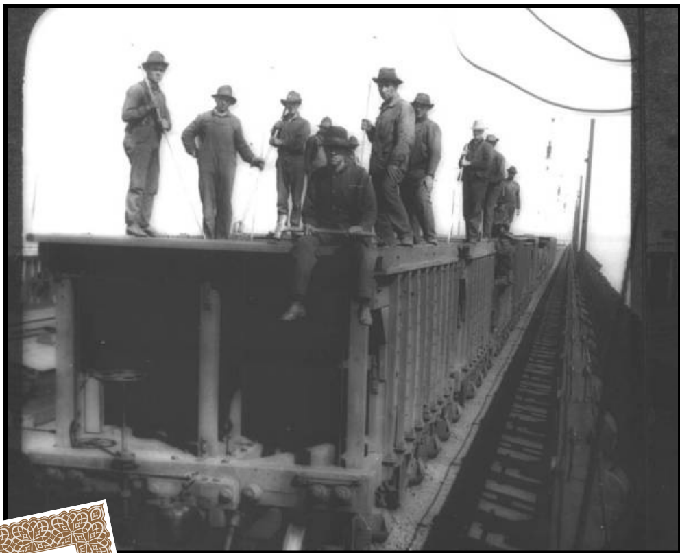
Workers dump the contents of a 50-ton ore car into the pockets of the Ore Dock in Escanaba, 1930. Original held at Northern Michigan University Archives.
