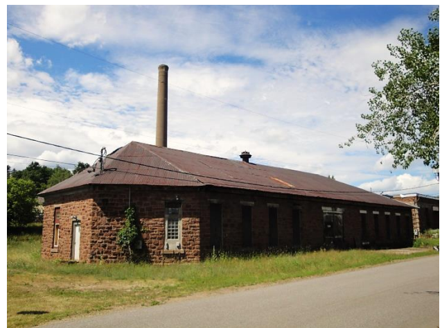
Hamilton Mine Sandstone Buildings, July of 2013
