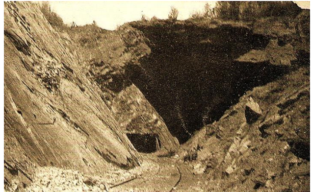
Entrance to the Quinnesec Mine, ca. 1906
