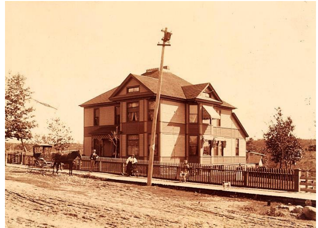
Pewabic Mine Hospital and Home of Dr. James Ashley Bangs, 837 East B Street, ca. 1893-1900
